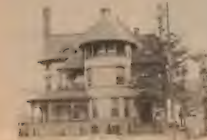
IN 1885, Eber Culver designed and built this three-story castle-like Richardsonian-Romanesque-style home. The building now contains apartments -- like other one-time mansions on Millionaires' Row.
